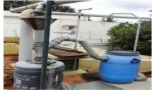
Fig.16. Roof top rain water harvesting
